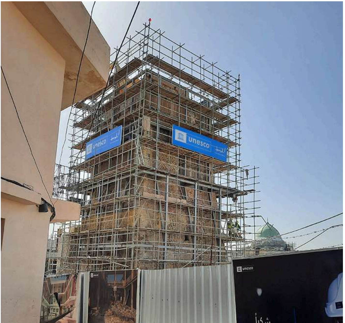
Mosul's iconic leaning tower minaret is under restoration.
